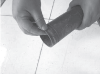
1. Before installation, whether the groove meet the standard should be checked and then wipe away the pickles, iron rust, greasy dirt on gasket ring and pipe.
