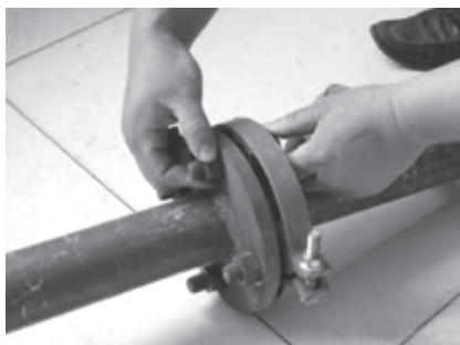
8.Insert standard bolts in the mated flange holes and screw nuts on them.
