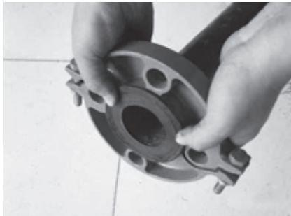
5.Assemble gasket in the pipe ODand flange groove, to keep the gasket in right orientation.
